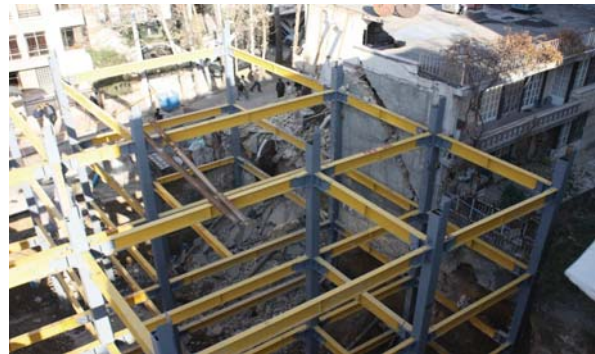
IOM Building Earthquake Resistance Assessment
