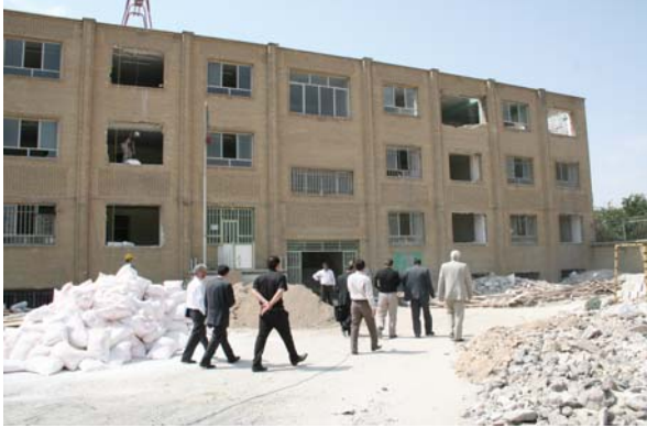
Seismic retrofitting of a school building, Tehran.
